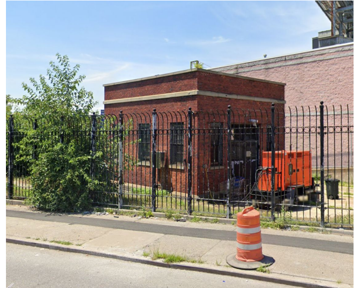
19 th Street Pump Station, constructed 1951
